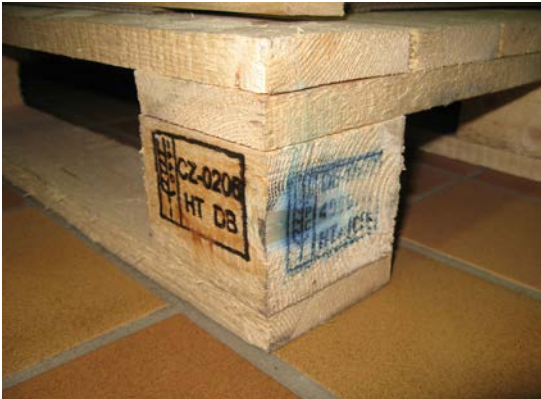
Two different ISPM 15 marks on one pallet block
