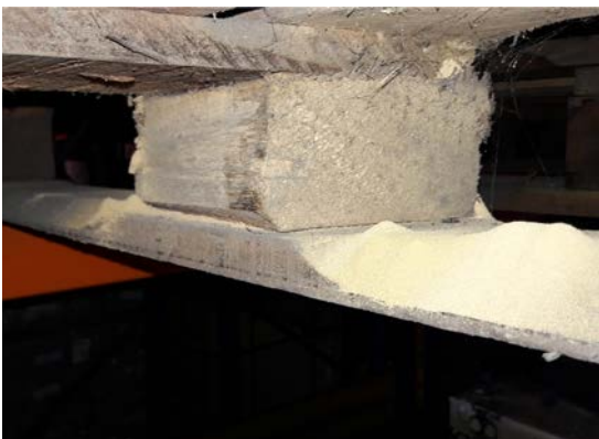
Fresh sawdust and wood residues may be a sign of an active insect infestation
