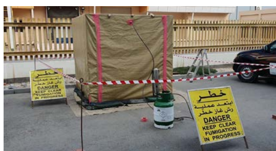
Fumigating wood packaging material in Bahrain
