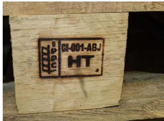
Second hyphen in producer/treatment-provider code
