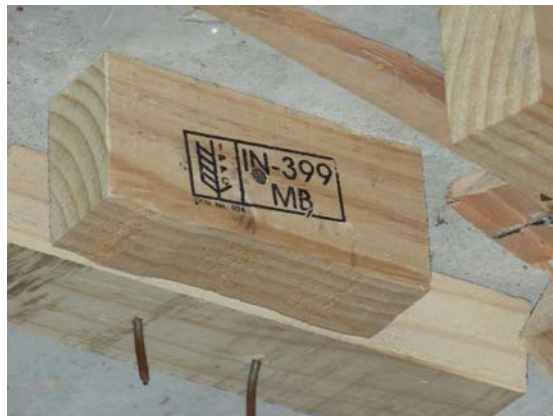
Treated wood dunnage that has been marked after it has been nailed in place
